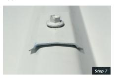
8 Barge capping needs to accommodate the slight rise in the joint area.
