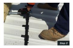
4 Position the MonoLap® roof lap joint roll with the centre of the hole in the protruding nylon part over the centreline of the support, and the foam further away from the higher end of the lower sheet.
