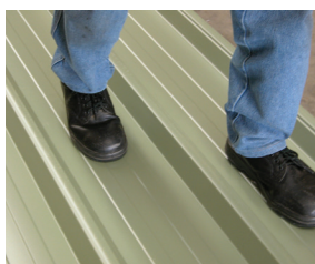
Walk only in pans, or on ribs at purlin supports.
