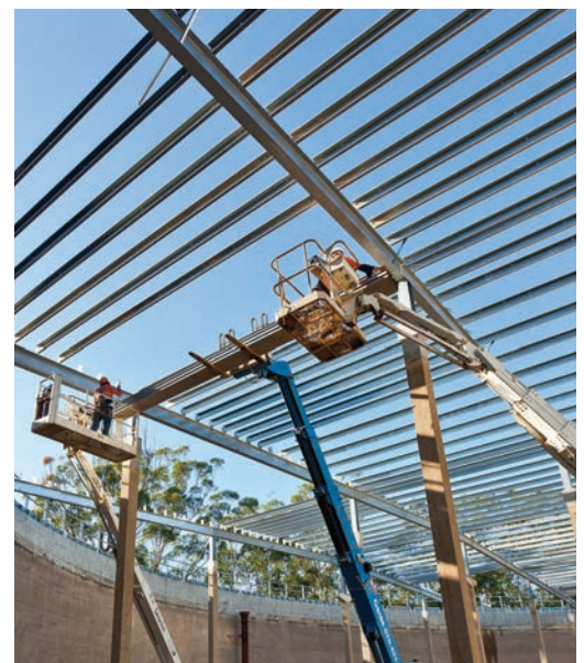
ZAM® purlins used for roofing of water reservoir ▲
