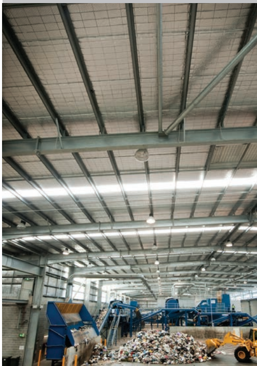
ZAM® roofing purlins at waste recycling centre ▲
