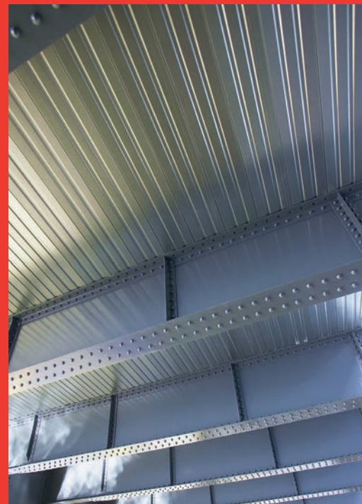
ZAM® formwork on river footbridge ▲
